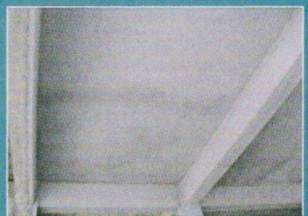
Expose finish with painting
