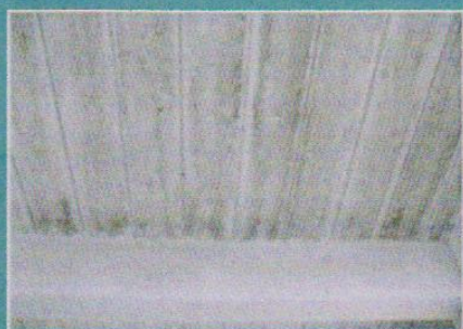
Soffit of slab after pointing with cement mortar
