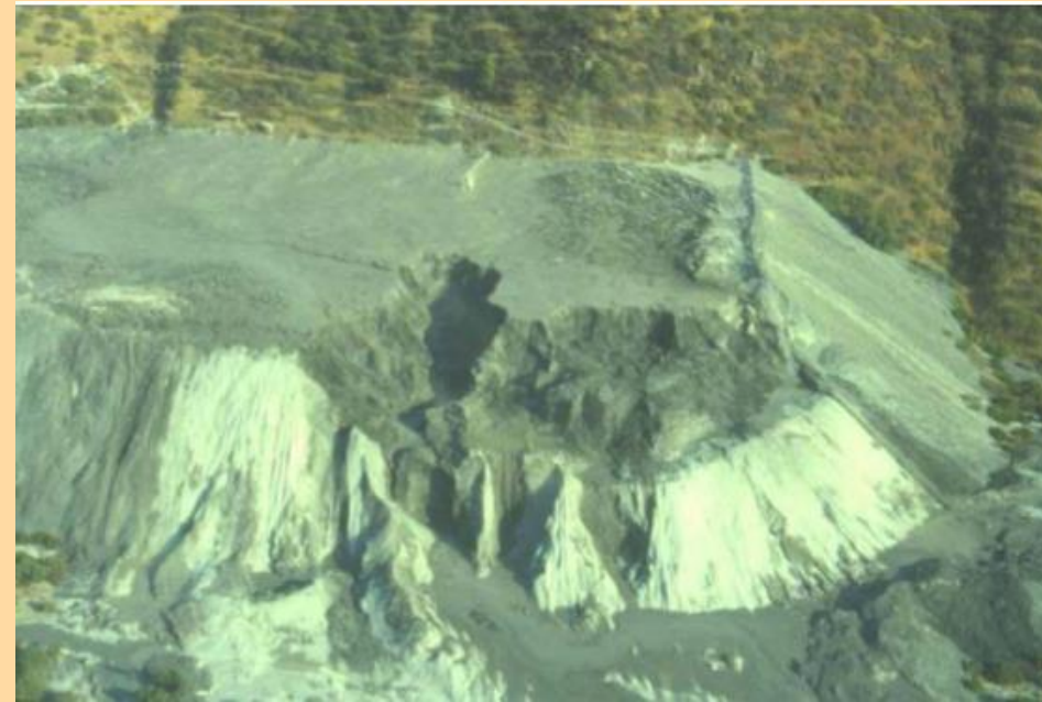
Failure of Cerro Negro Dam Chile Earthquake, 1985
