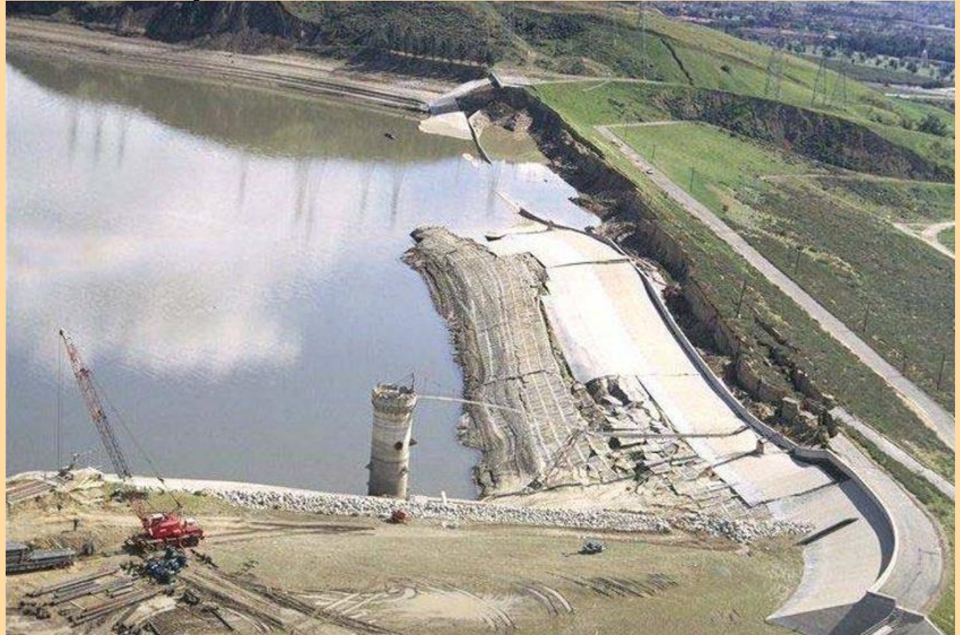
San Fernando Dam after Earthquake, 1964
