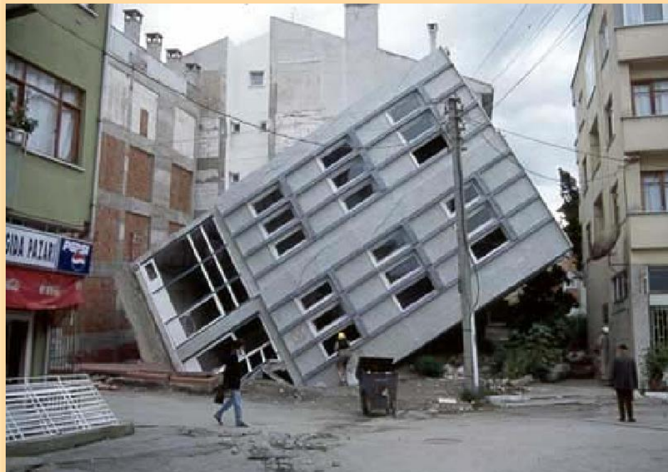
Mariana bay, USA, Loma Prieta Earthquake, 1989
