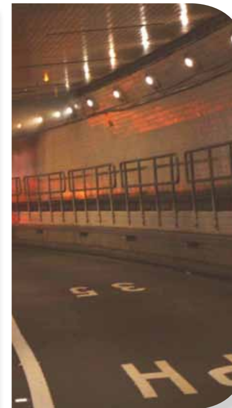
< Figure 5 - Photography of the fire tests in the Lincoln Tunnel
