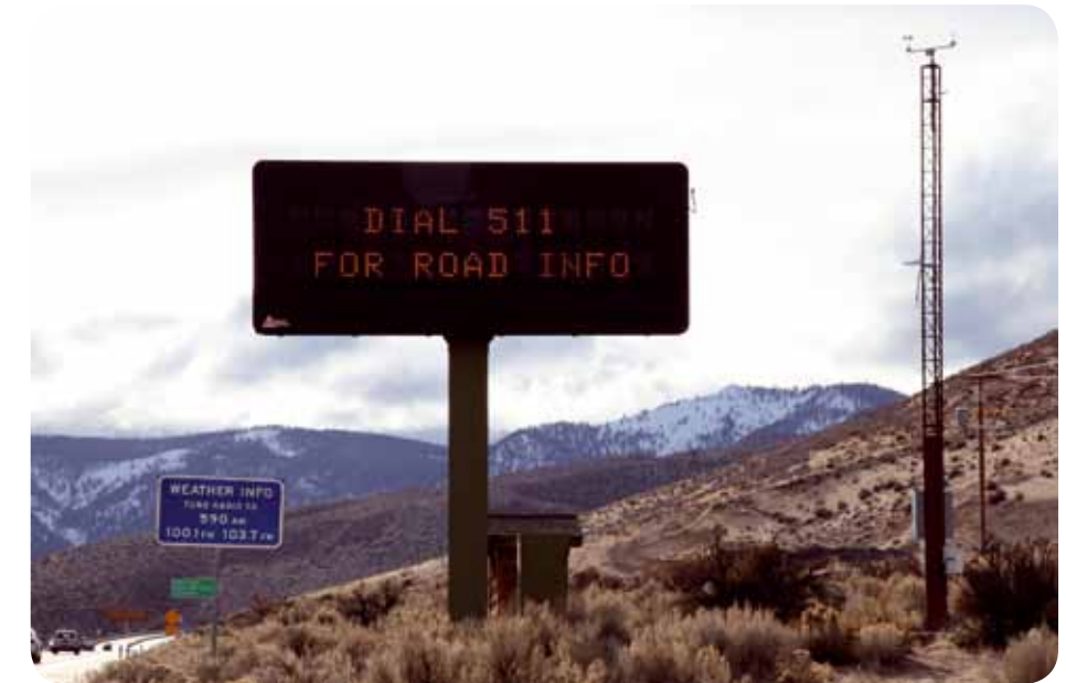
Figure 2 - RWIS collects roadway conditions and Dynamic Message Signs communicate conditions to users.
