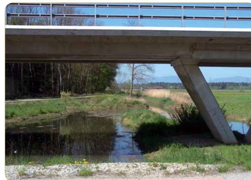
*Figure 4 - The T10 between Morat and Neuchâtel cuts through important wildlife corridors. Appropriate mitigation measures such as this bridge replacing a culvert were taken (photo courtesy of Marguerite Trocmé).*
