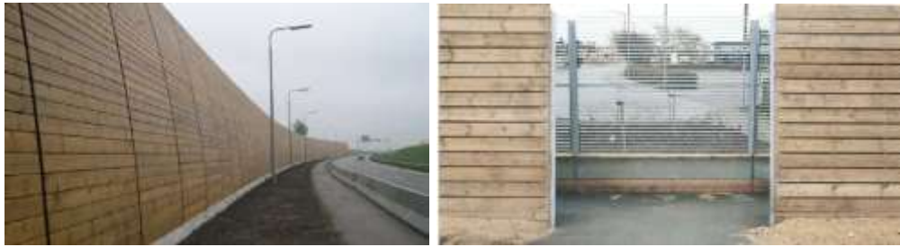
Figure 6.8 Examples of wooden acoustic barriers installed in Europe; [57].
