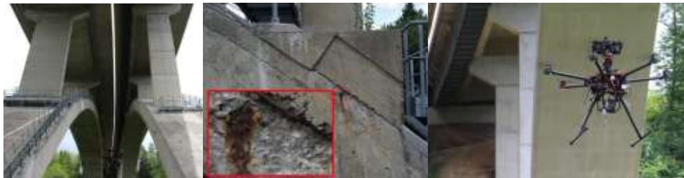
Figure 4.7 Inspection of an arch bridge by a drone; ASFINAG, Austria.
