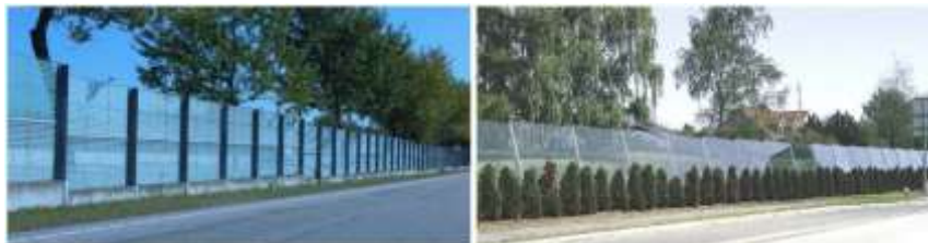
Figure 6.9 Examples of translucent barriers in Denmark; [57].
