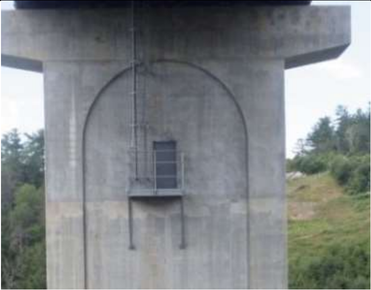
Access ladder and door detail.
