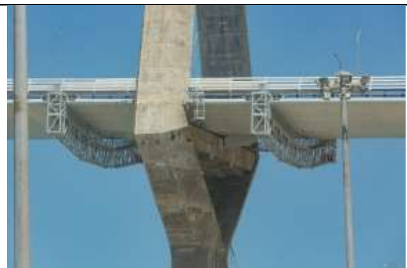
The platforms originally used during the construction of the cable-stayed spans of the bridge, for welding operations and others, were maintained as permanent moveable platforms.
