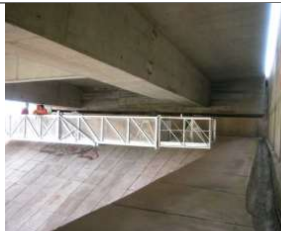
Description for platforms, landings, walkways, catwalks, etc.: walkway along retaining wall between abutments.
