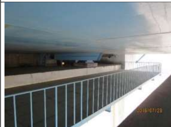
Item i: Bearing inspection platform.
