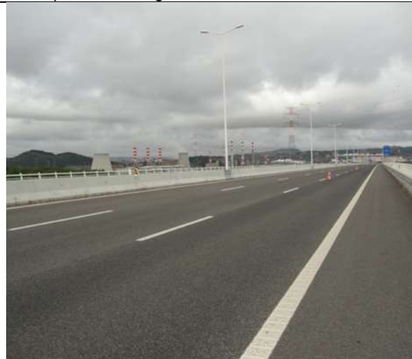
Lighting provided in central reserve which permits use of under bridge inspection vehicle.
