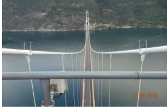
Railings on both side of main cables. Latchway system installed on railings.
