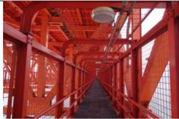
Item a: ---Inspection access platform.
