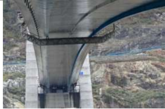
Access platform for outer surfaces box girder.
