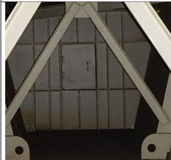
Interior steel hollow box girder painted white.
