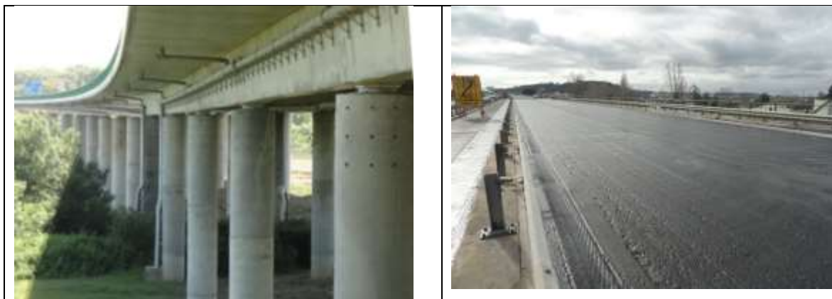
Top of piers adapted to receive platform for maintenance work on bearings.
