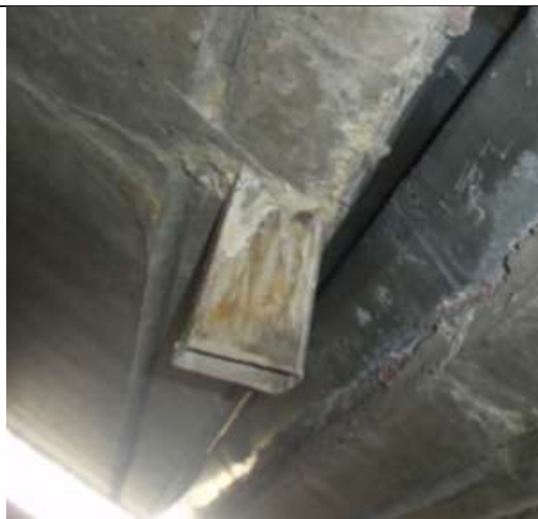
Expansion joint drainage.
