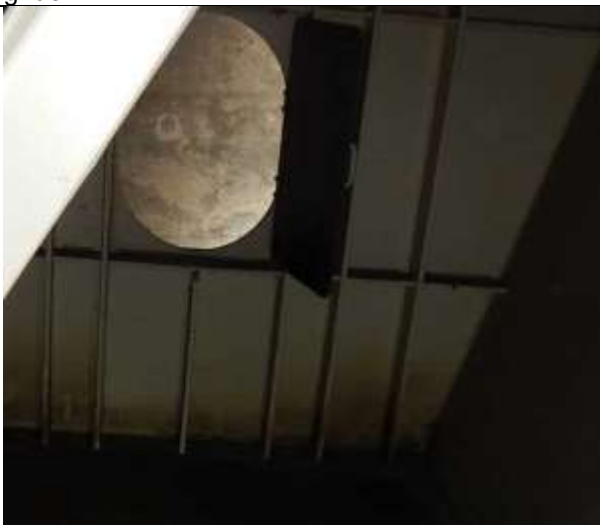
Interior steel hollow box girder painted white.
