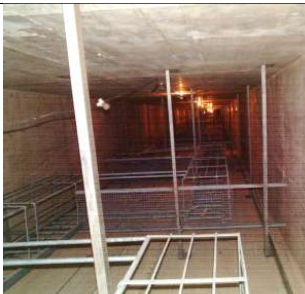
Ladder in the interior of the pier.
