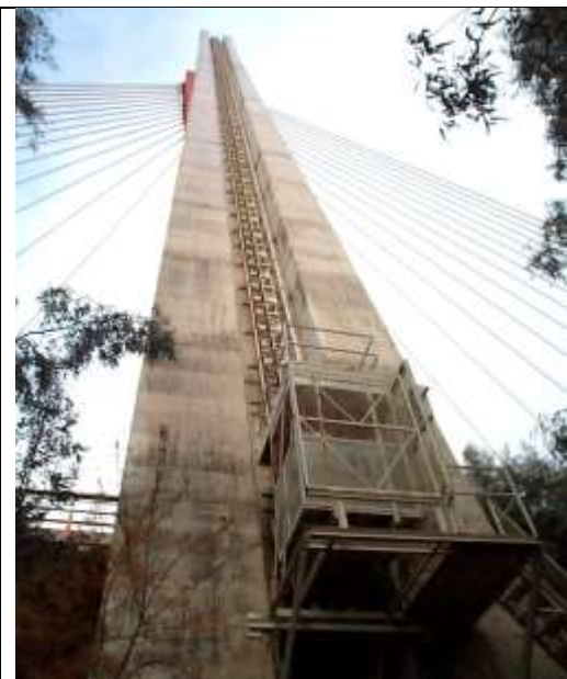
Lift on the exterior side of a pier.
