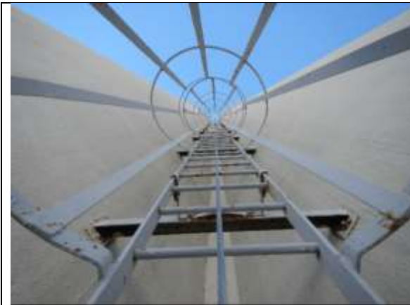
Item-f: Fall protection system at cat ladder.
