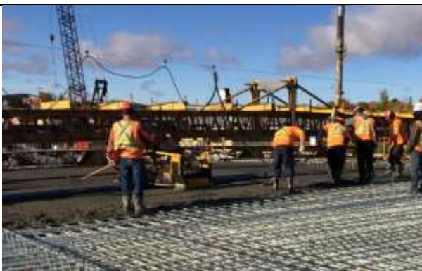
Concrete machine used for finishing surface of bridge decks.
