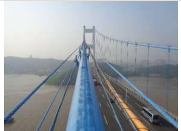
Item e: Main cable inspection walkway.
