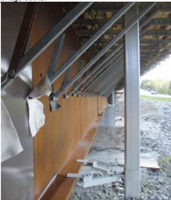
Deck scupper extends beyond bottom level of girder.
