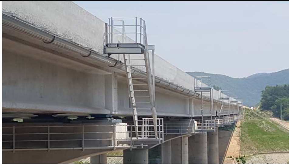
Walkway platforms around pier heads.
