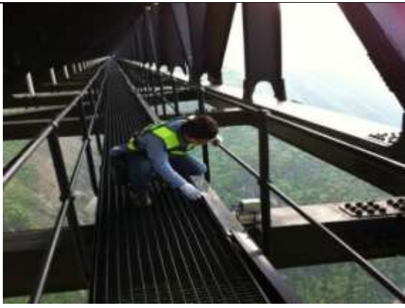
Item e; Truss bottom chord inspection access.
