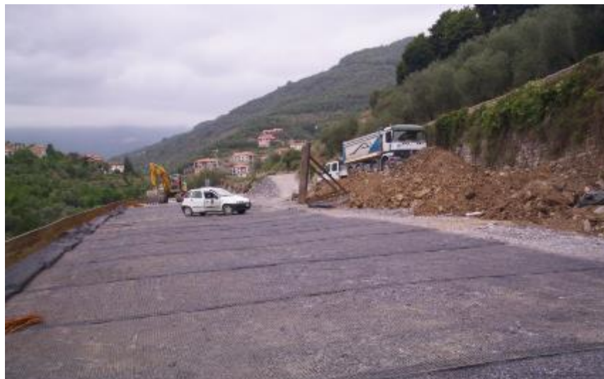
Figure 7.8: Geosynthetics for embankments.
