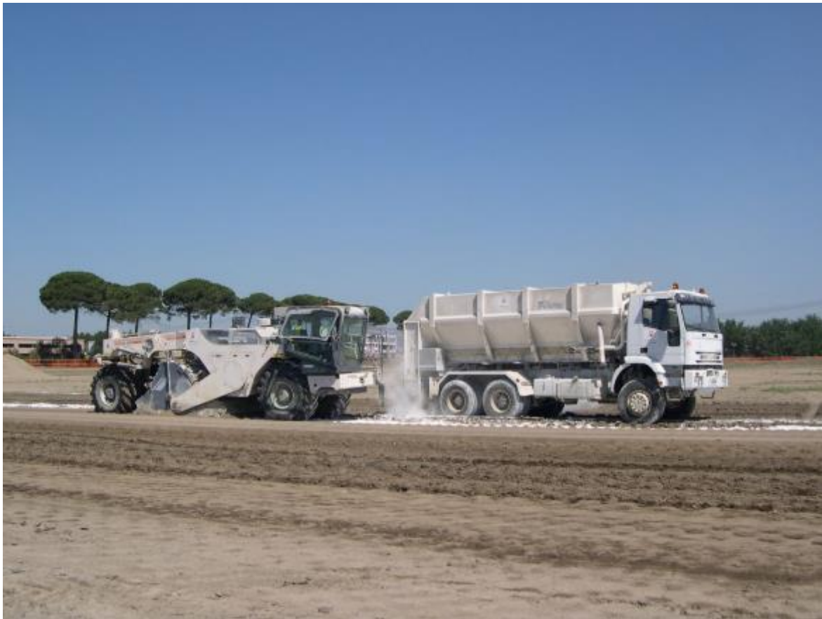
Figure 7.6: Pulvimixer for lime treatment and feeder
