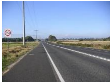
Figure 2.17 Shoulder Sealing, Source: iRAP
