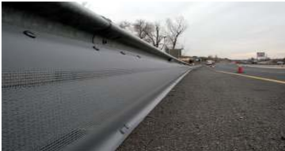
FIGURE 11 : MOTORCYCLIST PROTECTION SYSTEM (MPS) FITTED TO THE EXISTING BARRIER SYSTEM
