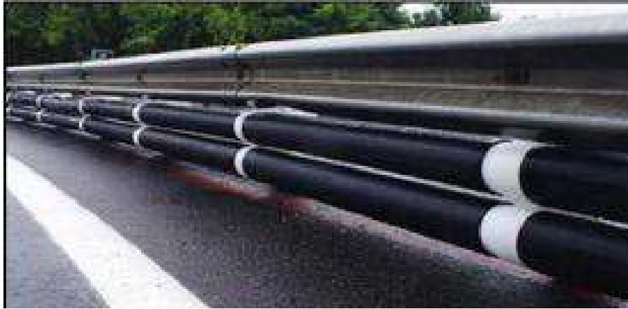
FIGURE 10 : PHOTOGRAPH OF "MOTOTUB " FITTED TO EXISTING BARRIER SYSTEM
