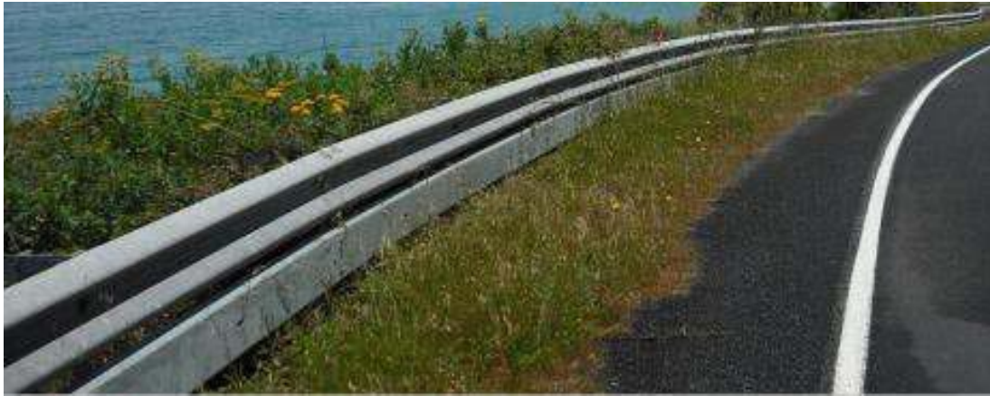
FIGURE 8: PHOTOGRAPH OF RUB RAIL FITTED TO AN EXISTING W-BEAM Source : Safe Direction
