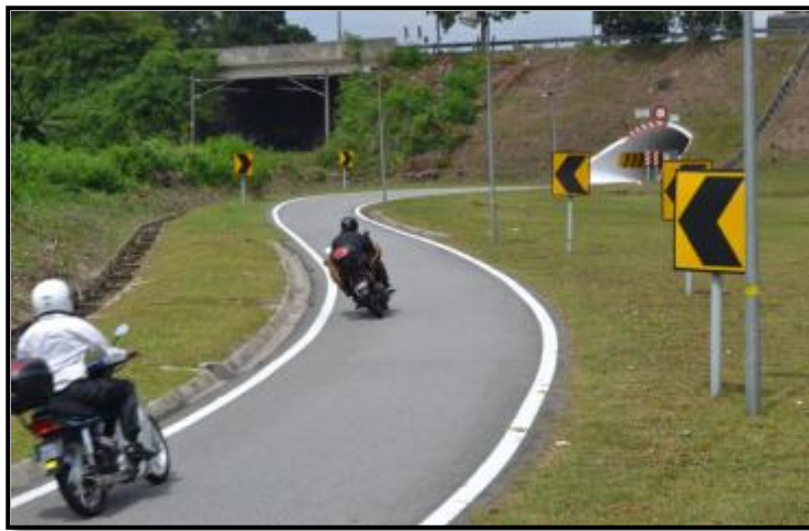
FIGURE 4 : AN EXAMPLE MEANDERING ALIGNMENT BEFORE ENTERING UNDERPASS
