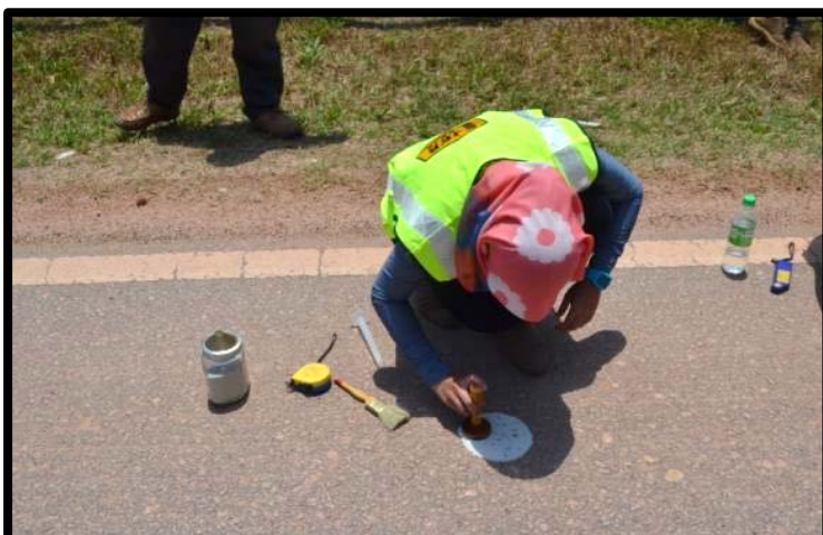
Picture 3: Mean Texture Depth Being Measured At Site.
