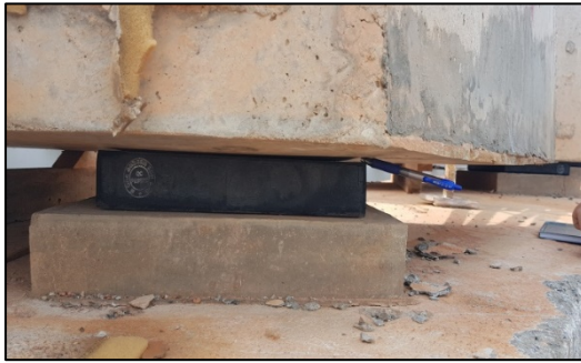
Figures 6 (a) : Position of base of precast beam, rubber bearing and concrete pedestal
