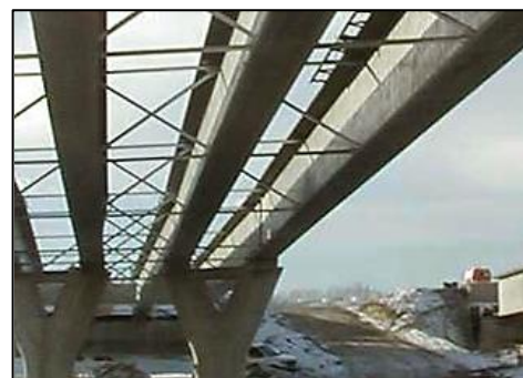
Figures 3 (b) : bracing system by using steel member erected in between beam
