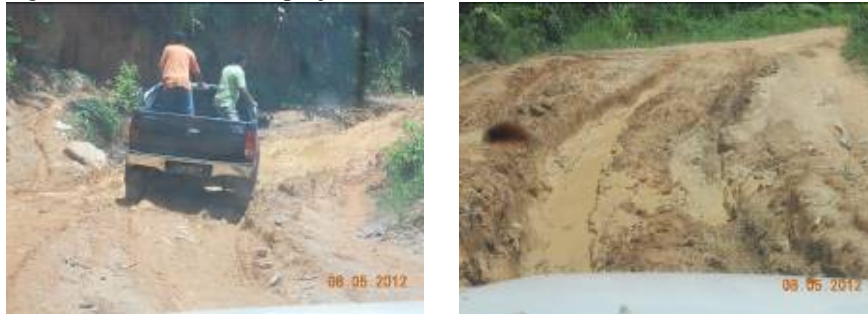
Figure 1: Condition of existing road before construction.
