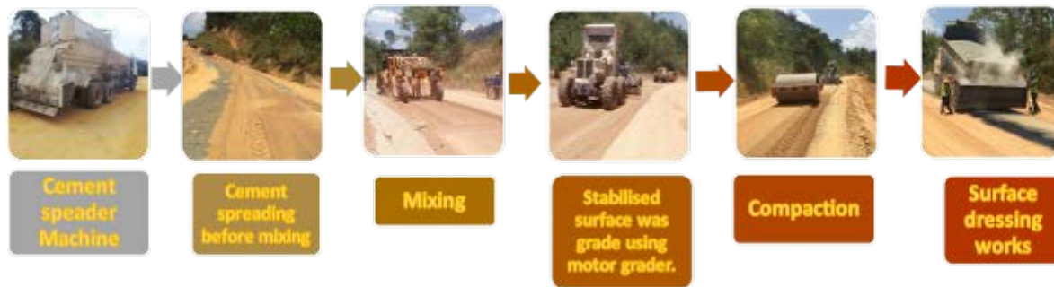
Figure 7 : Soil stabilisation process
